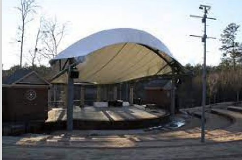
Lakeside Amphitheater Along Lakeside Trail, next to the Shi Center for Sustainability
